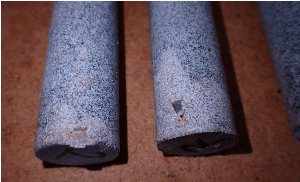
Picture 2: Detail of damage of coating at dowel No. 2 (about 4mm x 1mm) and dowel No. 7 (about 3mm x 6mm).
